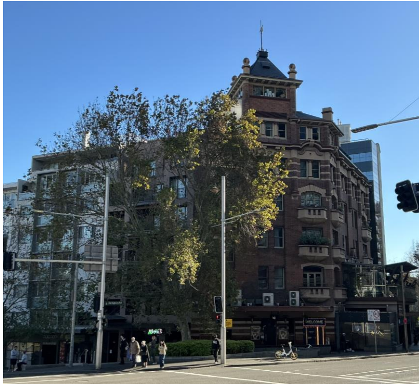
Figure 1: 244-248 William Street, Potts Point, viewed from the south-west
